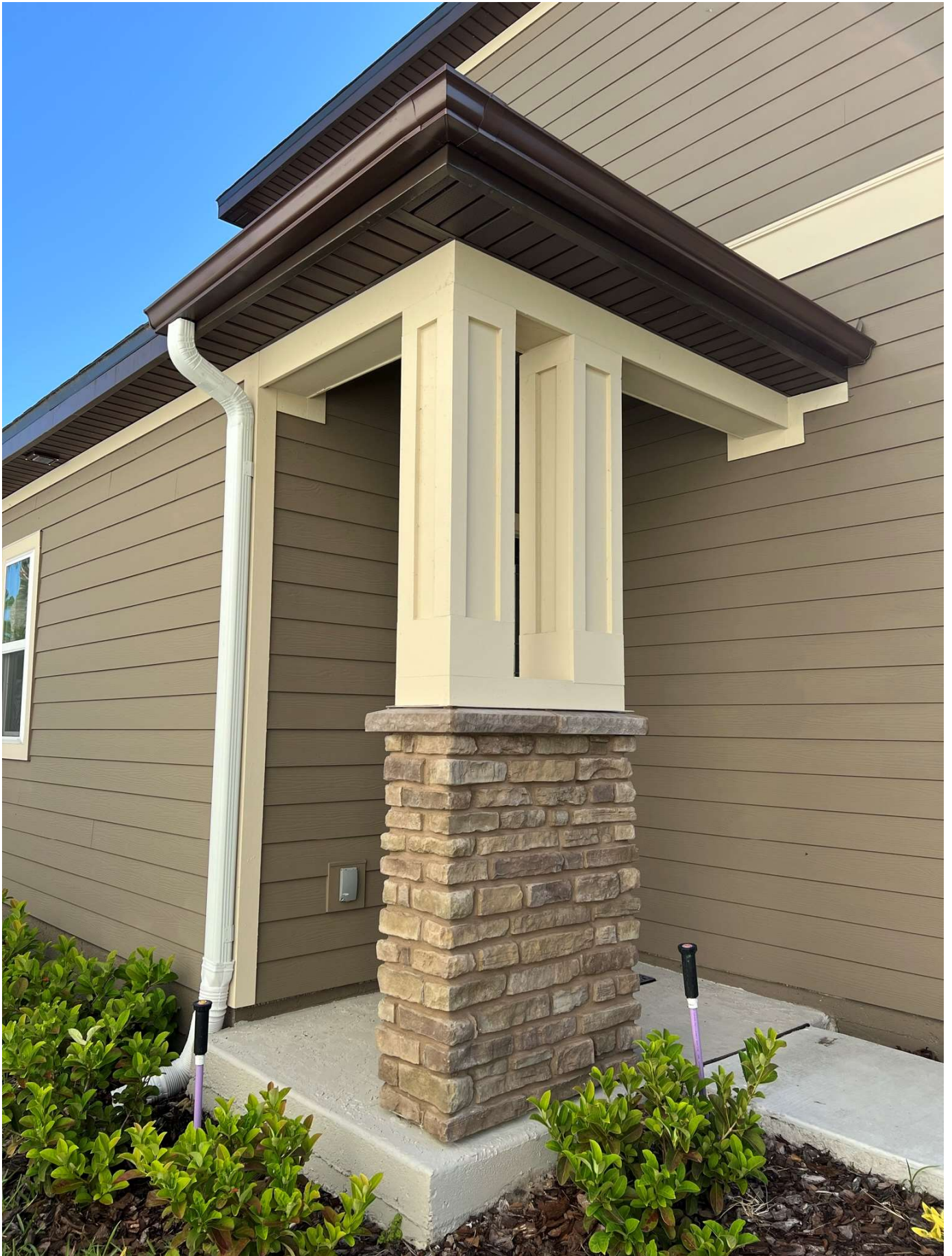
Front porch with rain gutter.
