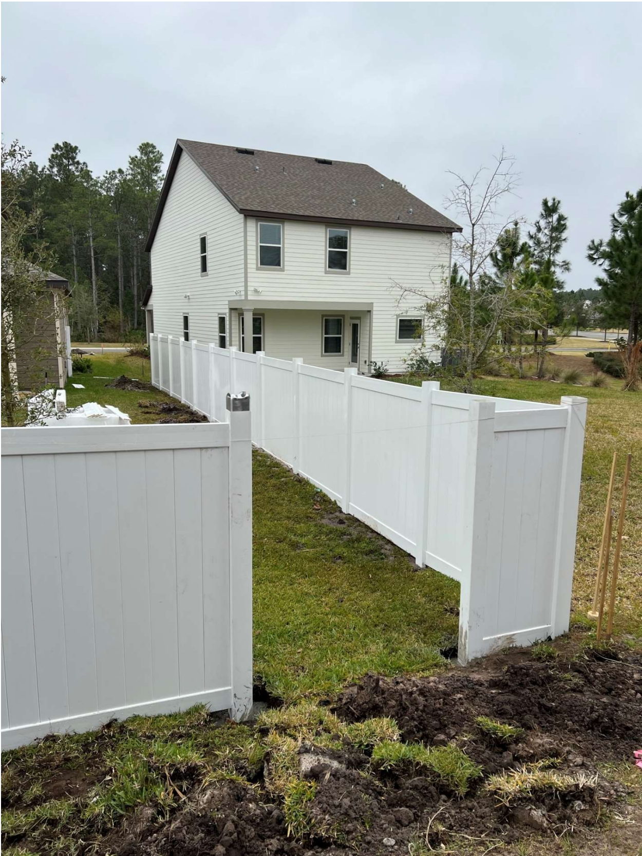
These posts use a lot of concrete.
