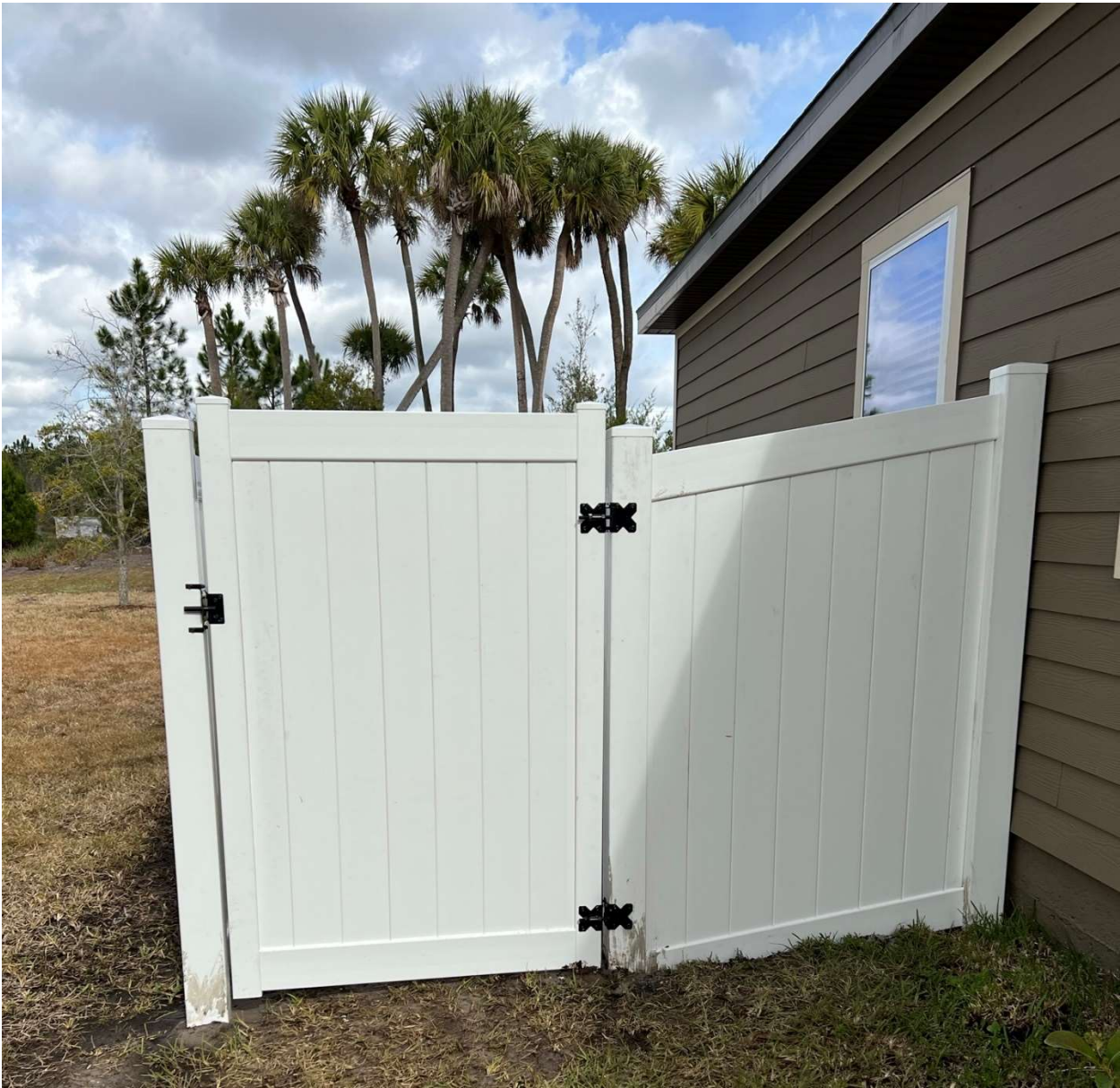
Finished gate on right side.
