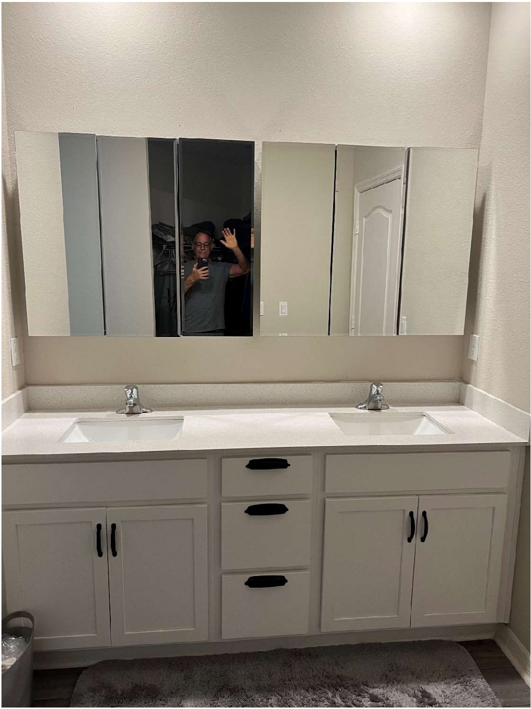
The 2 mirror cabinets installed in the MB Bathroom.
